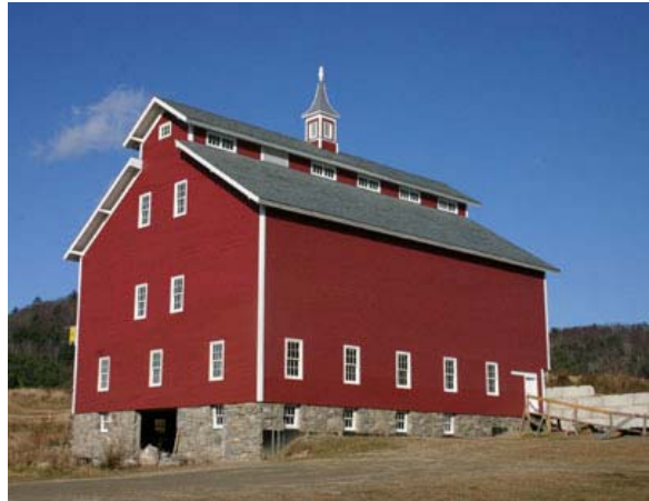
The historic West Monitor Barn as it appears today
